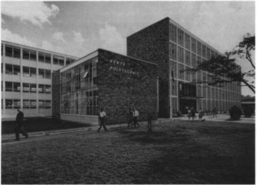
PLATE 22.3 Above: biology laboratory in a College of Education, University of Lagos, Nigeria, 1968; below: the Kenya Polytechnic and Technical Institution, 1968
