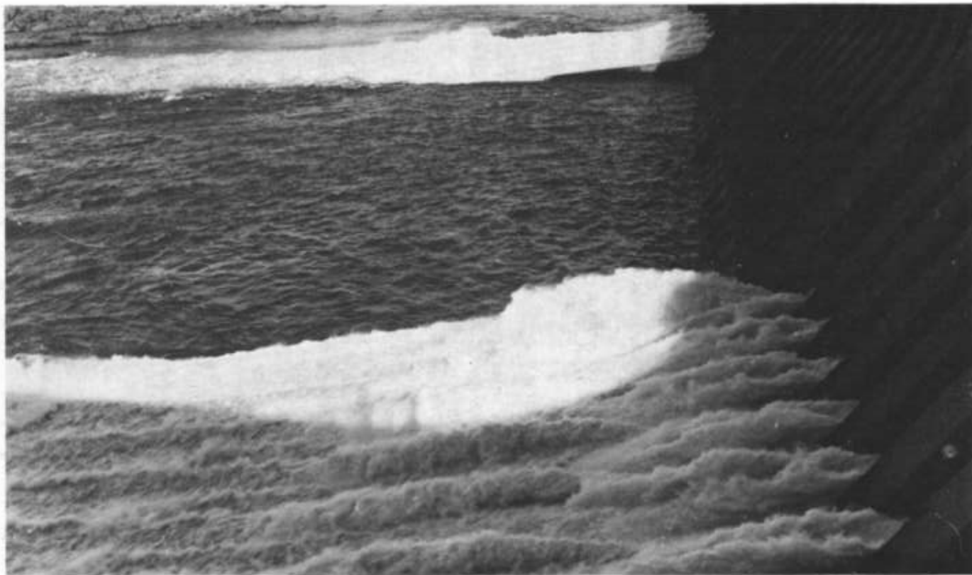
PLATE 17.1 The Aswān dam (Egypt) in 1937
